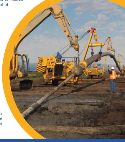
Installing new pipe into a horizontal directional drilled pilot channel
